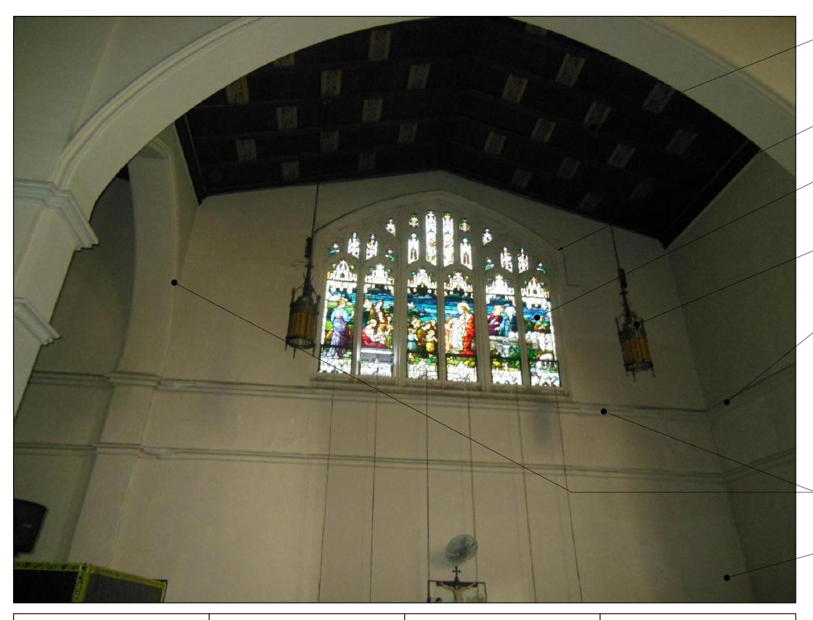
CONTRACTOR TO PROTECT EXISTING PAINTED WOOD CEILING, WHICH IS TO REMAIN, THROUGHOUT CONSTRUCTION SCOPE. IF ANY FINISHED WOOD IS REQUIRED TO BE REMOVED AS A RESULT OF INTERIOR SHORING OR STUCCO FINISHING THE CONTRACTOR SHALL CAREFULLY REMOVE, SAVE FOR RE-SETTING AND INSTALL AT APPROPRIATE STAGE OF WORK SCOPE COMPLETION. ANY EXISTING DETERIORATED WOOD SHALL BE BROUGHT UP TO THE ATTENTION OF THE ARCHITECT.
